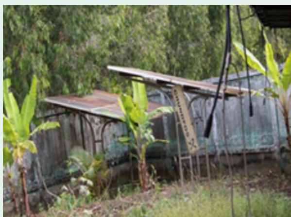
THE PANEL ARE RUSTED, PEELED
