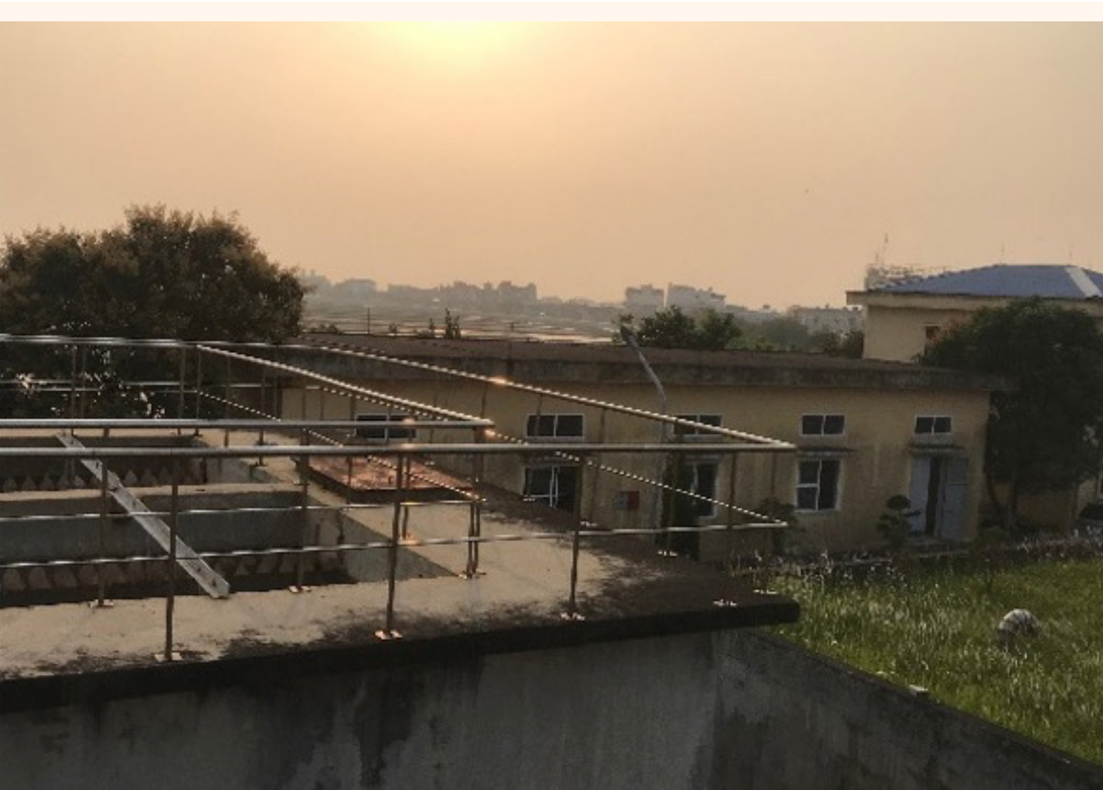
Water plant Giao Thuy, Giao Thuy district, Nam Dinh province
