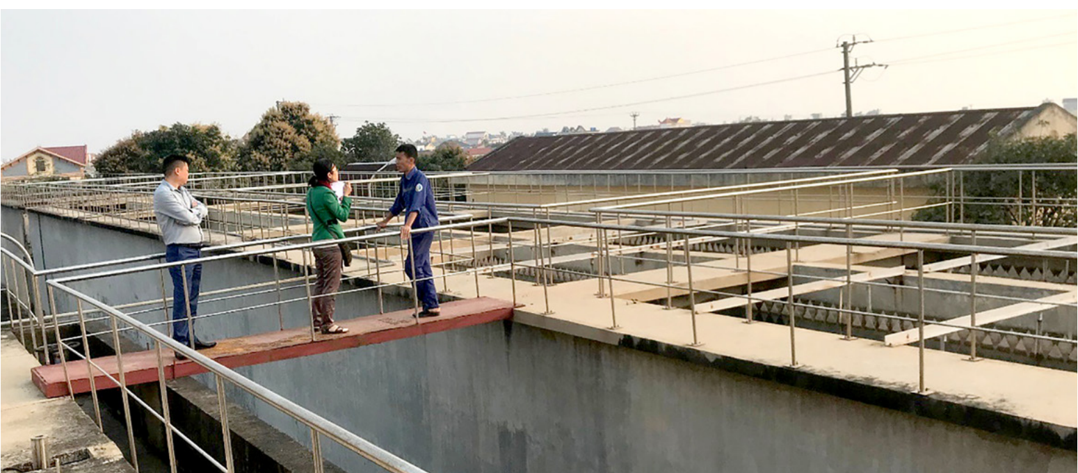
Filtering tank at water plant Giao Thuy, Nam Dinh province
